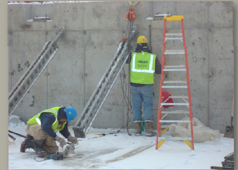
Image provided by Mabey Bridge & Shore, Inc
