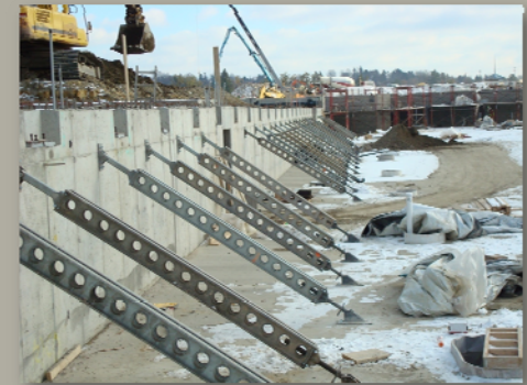
Image provided by Mabey Bridge & Shore, Inc
