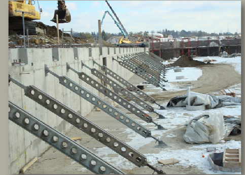
Image provided by Mabey Bridge & Shore, Inc
